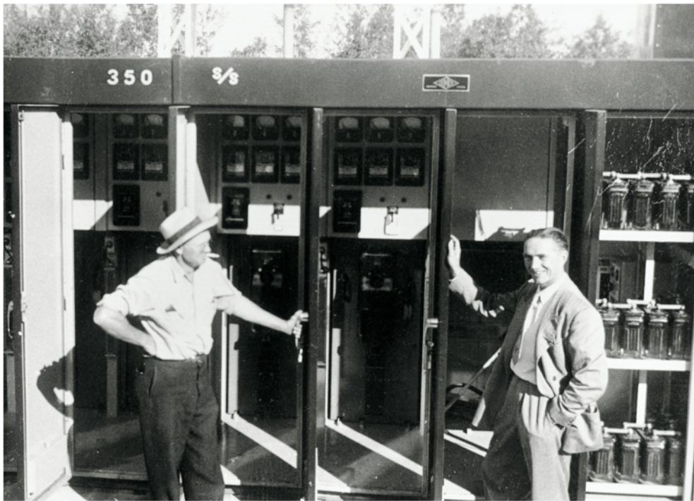
ABOVE: Roy Fitzsimmons (left) and Stan Hampton (right) at 350 Substation.
