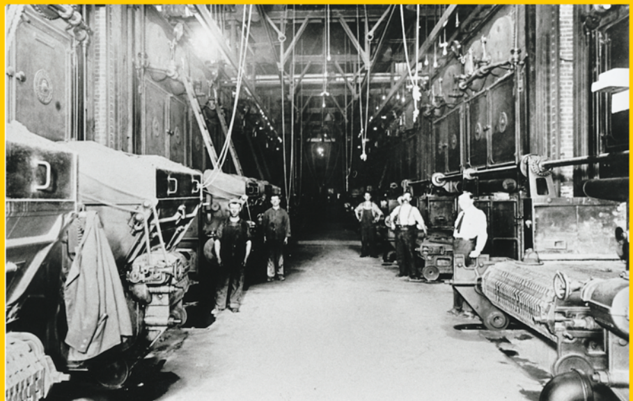
BELOW: Chain grate stokers used with a boiler installed in 1914. Cunningham is in the right foreground wearing a white shirt and tie.
