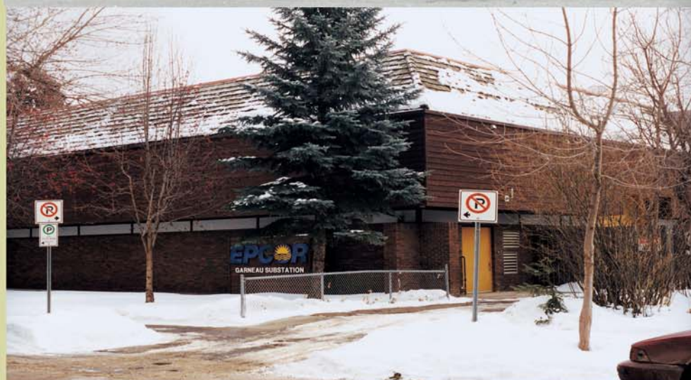
TOP RIGHT: An example of early substation design: 600 Substation on 124 Street.
