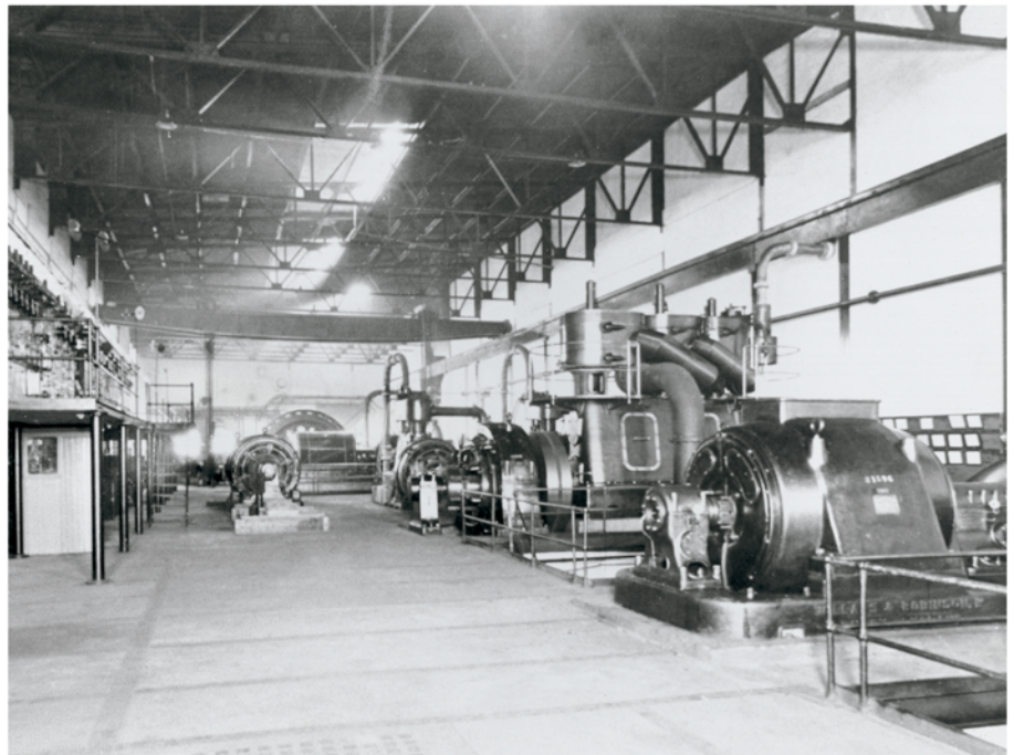
RIGHT: Inside the Rosedale plant in the 1920s. The tallest unit is the 750 kW triple expansion and engine, installed in 1910 and removed in 1949.
