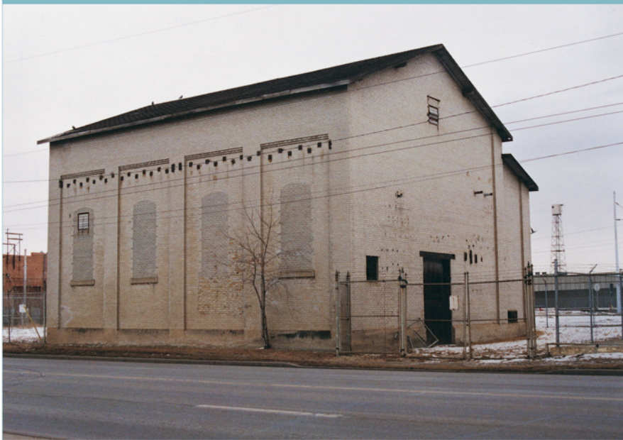
LEFT: 100 Substation in 2000.
